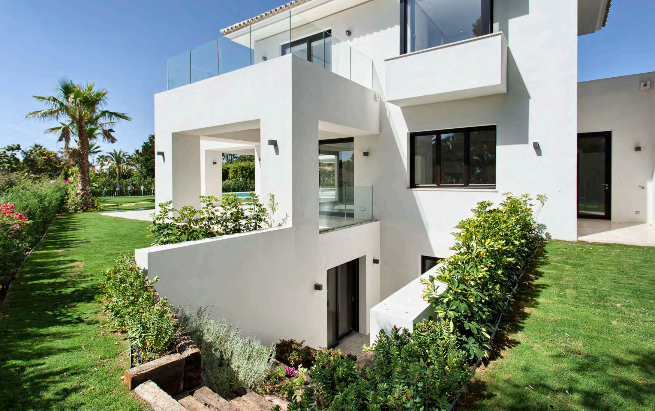
The Entrance to the Ground Floor
